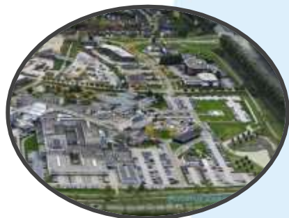
Hospital Waste Water Sneek
