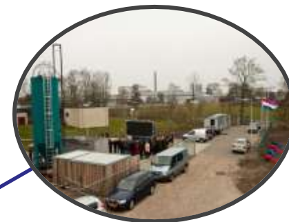
Municipal Waste Water Wetterskip Leeuwarden
