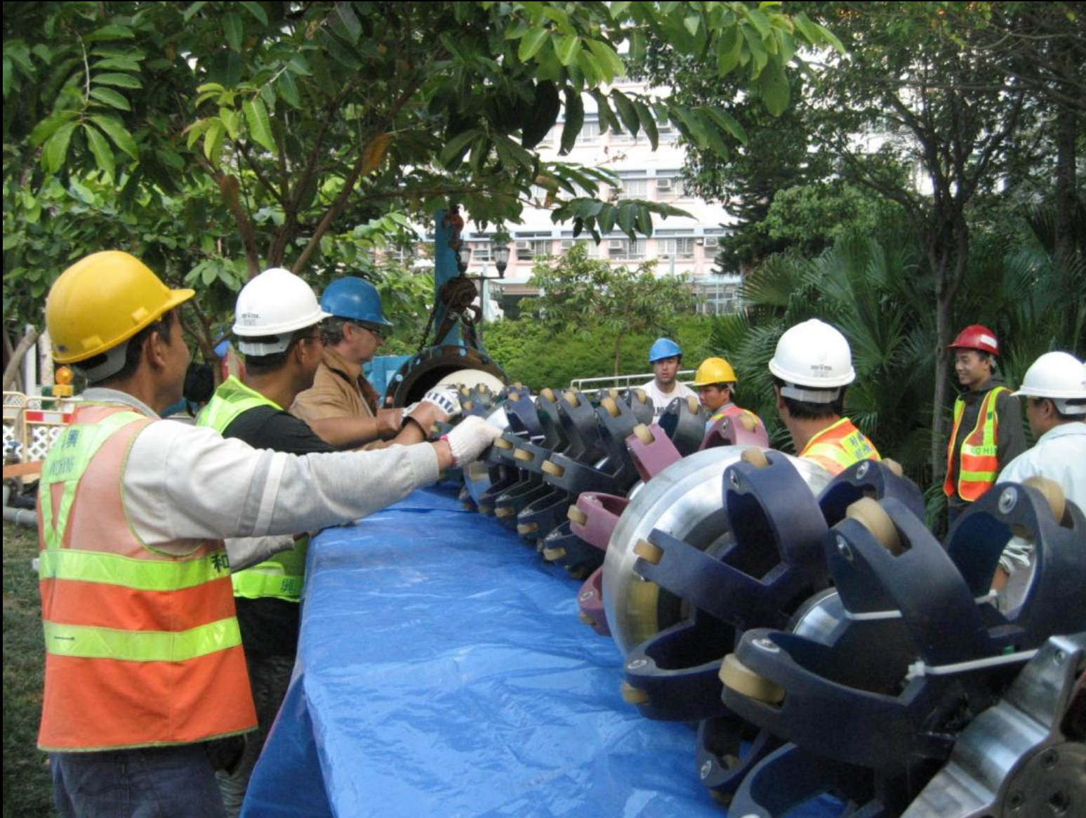
A SeeSnake Tool is prepared for launch into a Potable Water Main in Hong Kong Dec 2010
