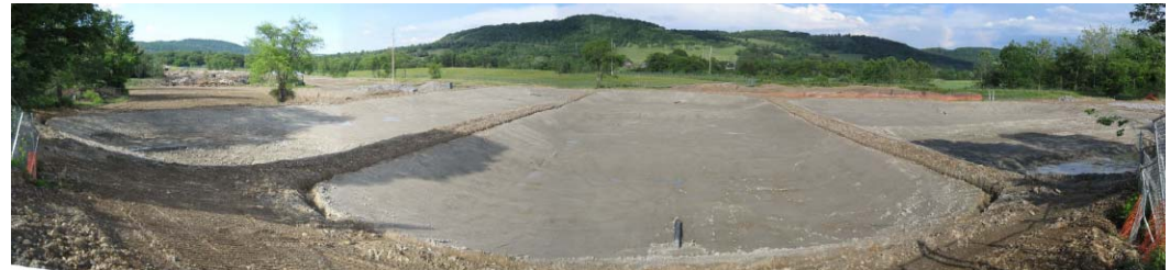
Wellsville, New York Engineered wetland petroleum hydrocarbon remediation project for BP (1,090 m 3 /day)
