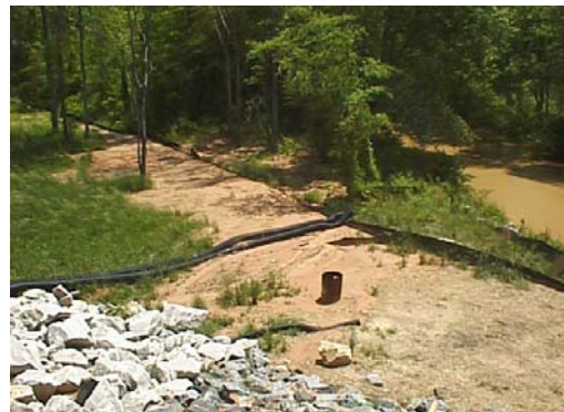
Figure 2: Result of poor soil stabilization
