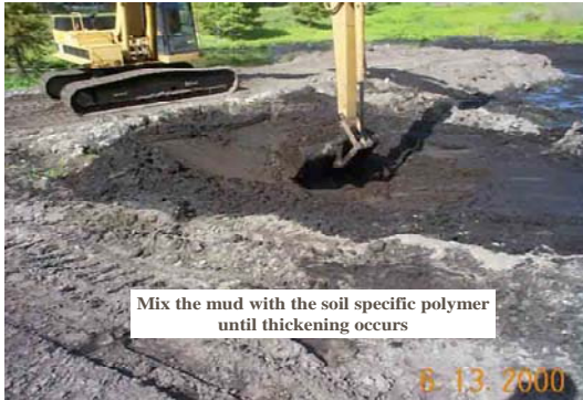
Figure 17: Mud mixing with polymer
